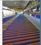
AUTOMATIC COOLING BED
